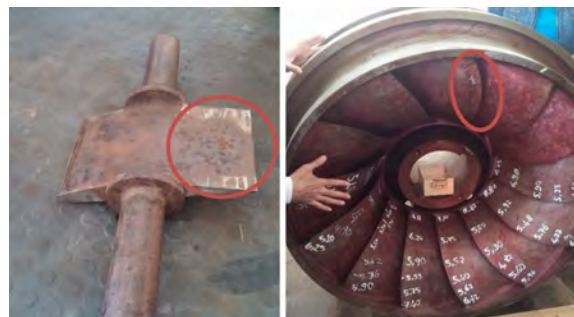
Figure 1. Picture of the existing guide vane and the runner
