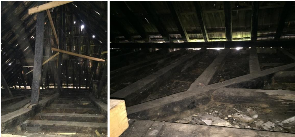
Figure 10. Roof structure of the Pozderac family house in Cazin (Ahmet Hadrovic, 2019)
