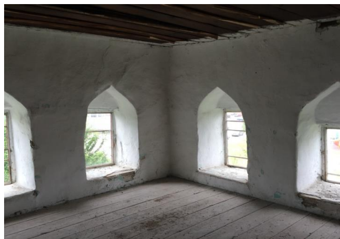
Figure 11. The Pozderac family house in Cazin: “large room” on the west corner of the ground floor (Ahmet Hadrovic, 2019)
