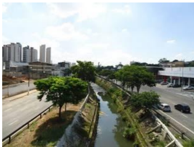
Figure 3 - View of the medium course towards the downstream. On the banks of the Ipiranga Stream are the lanes of Dr. Ricardo Jafet Avenue. Photograph: Amaral, 2018.
