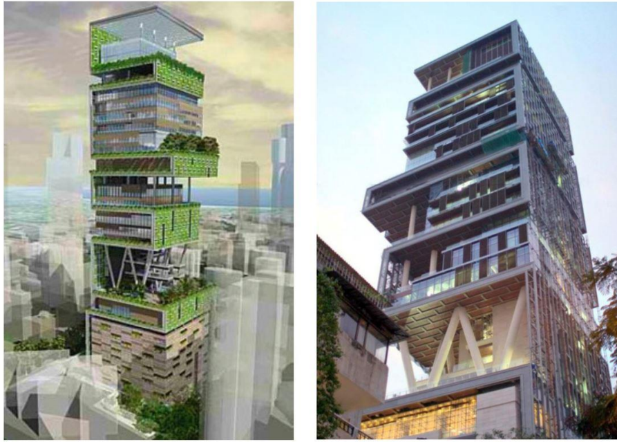
Figure 5. Application of Antilia Tower Project and 3d image of the initial project (Akkaya, 2019).
