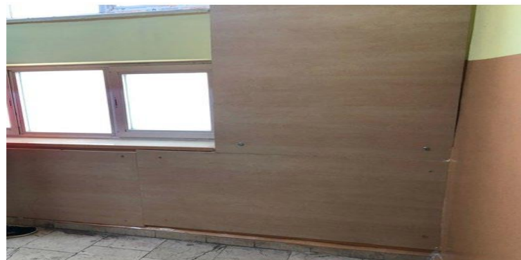
Figure 5. Precaution Taken for Structural Damage
