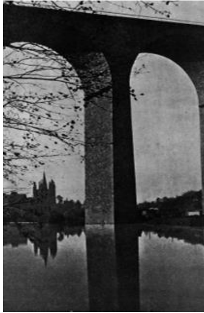
Figure 4. Paul Bonatz; Part of a Road Bridge [20]
