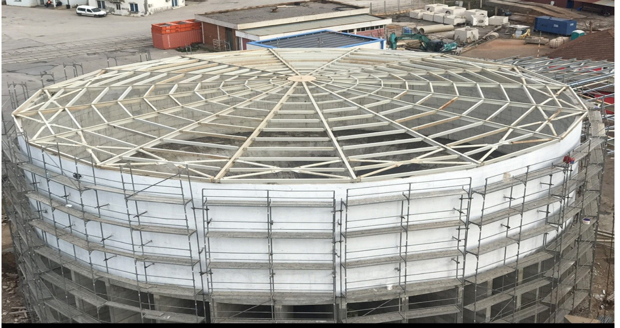
Figure 1. General view of the structure
