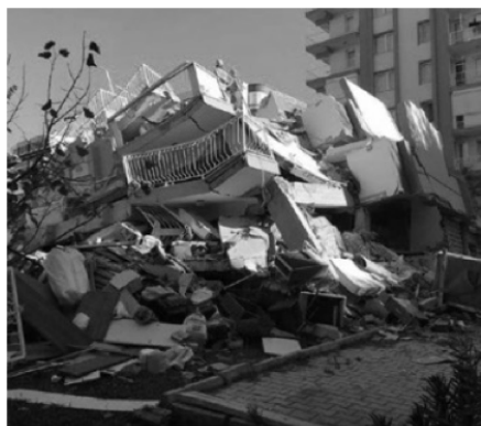
Figure 8: Collapse mechanism observed at the site (Photo from [10])
