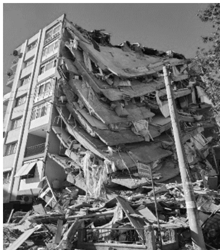
Figure 9: Partial collapse mechanism observed at the site
