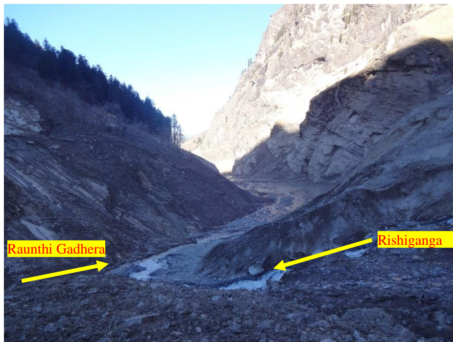
Figure 5: At the confluence of Raunthi Gadhera with Rishiganga where key damming was observed
