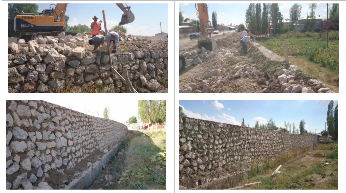
Figure 2: Photos showing project and construction sites
