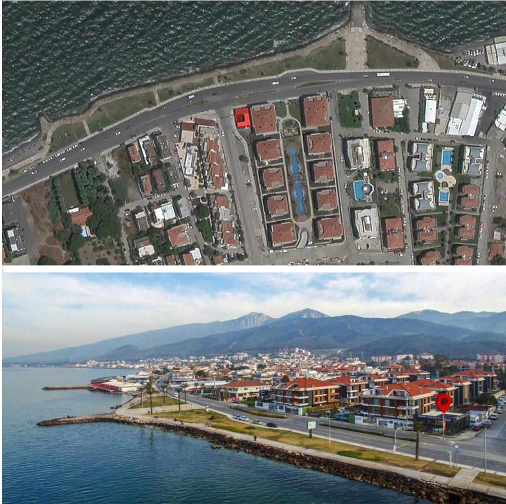
Figure 1 - Project site [Above: Satellite view; Below: Aerial view] (Photo credits: Çiçek Kardeşler İnşaat Ltd. Şti.)
