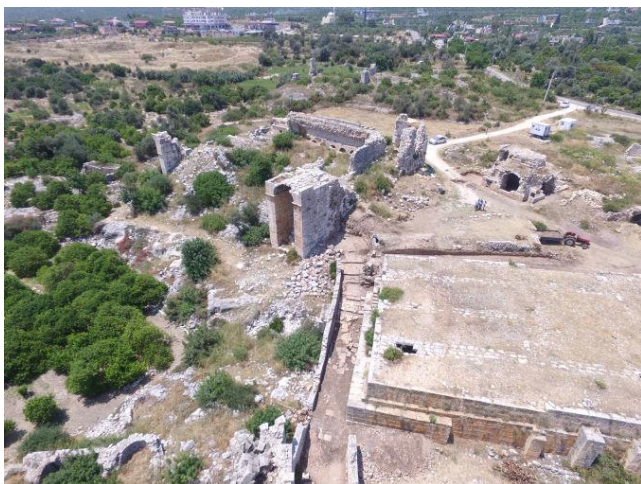
Figure 2. Akkale Cistern and buildings in Akkale
