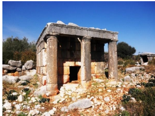
Figure 8. Roman period Monumental Temple constructed with isodom masonry technique in Kanlıdivane
