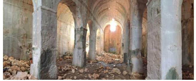
Figure 3. Interior view of Akkale Cistern
