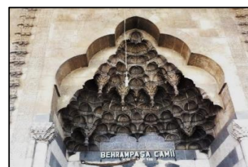
Figure 5. Detail of the muqarnas on the crown gate of Behram Pasha Mosque
