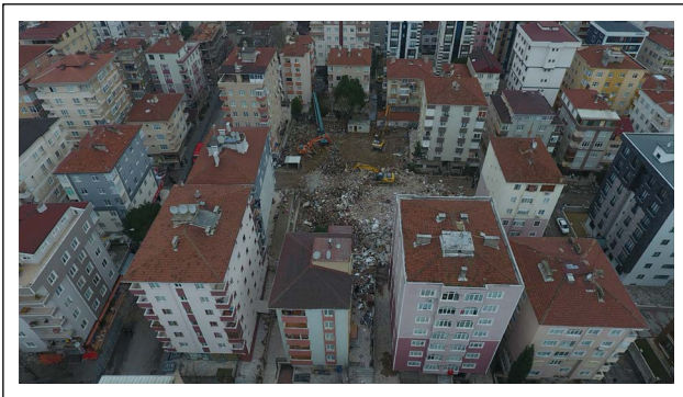
Figure 4. The view after removal of the wreckage of Yeşilyurt Apartment.
