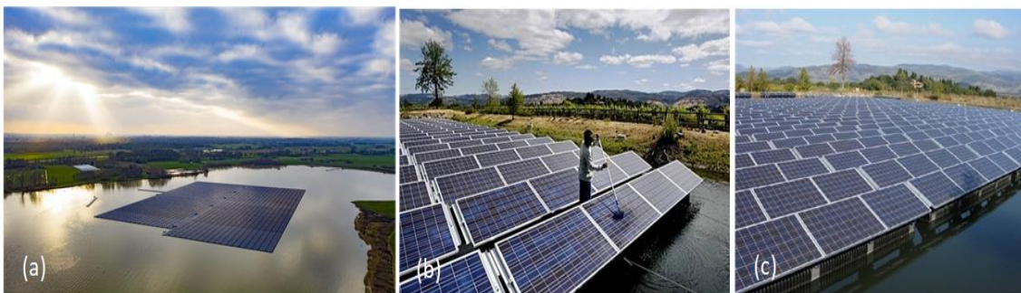
Figure 16- Aquavoltaic systems: (a) Floating PV plant on Dutch lake (PV TECH 2020), (b) Floating solar power system located in California's Napa Valley region (Solaripedia 2021), (c) India's largest floating solar plant (pv magazine 2021)
