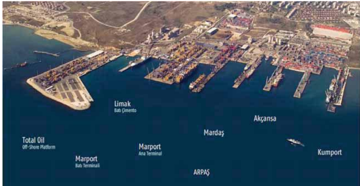
Figure 2. Facilities Directly Related to Ambarlı Port
