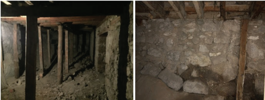
Fig. 19: Wooden pillars and stone walls in site B01. (By Karakuş, 2020)
