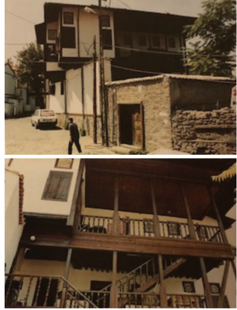
Fig. 6: A fine example of “hayat” in “Demirfirka” Neighbourhood “Doyran” Street (Tuncer, 2002, 53.)
