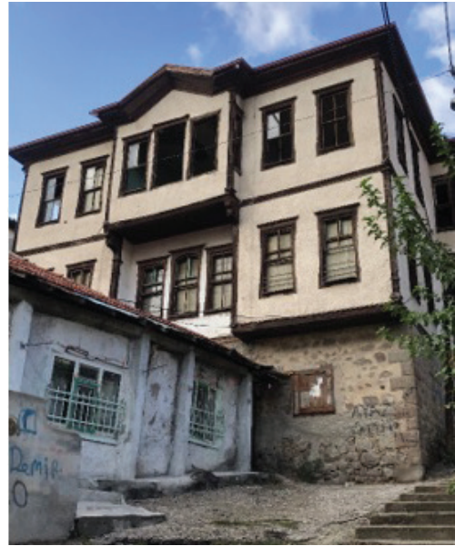
Fig. 7: View of Sadık Arslan’s House from Ulucanlar Street and Eryokuşu Street. (By Karakuş, 2020)
