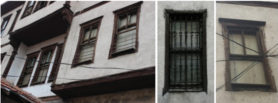
Fig. 38: Wooden guillotine windows and fence details of the building. (By Karakuş, 2020)
