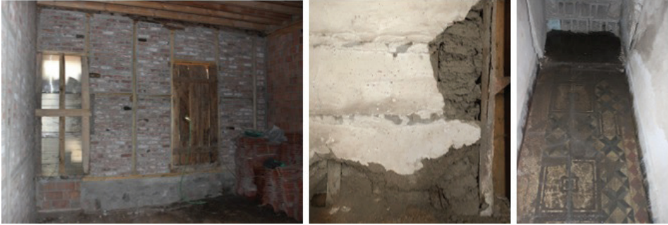
Fig. 20: Brick wall between wooden frames and original mud-brick wall in site Z03 and cement tile covering in site Z10. (By Karakuş, 2020)
