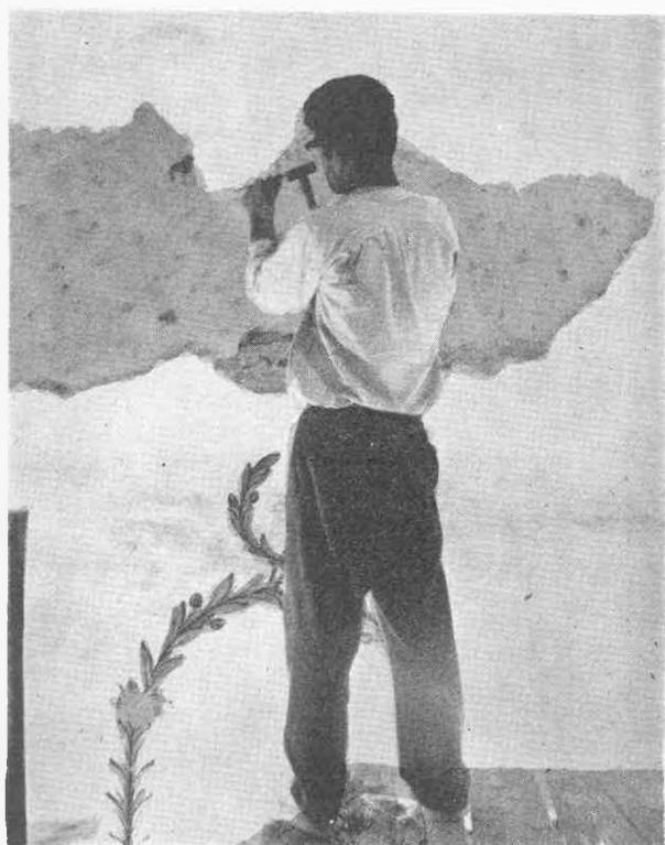
Plate 5 — Work in progress on the removal of plaster from the Cupola.
