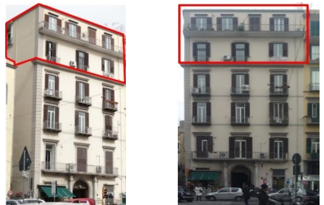
Figure 8. The facade of the building. In red the two floors probably added during the last two centuries
