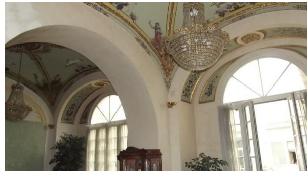
Figure 28. Photo of the sail vault on the first floor
