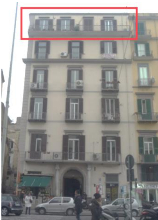
Figure 13. The main facade on the Riviera di Chiaia. In the red frame the last added floor made by r.c.
