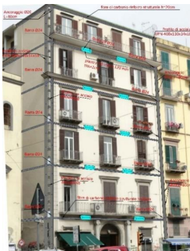
Figure 40. Rendering of some of the structural reinforcing on the external wall of the building
