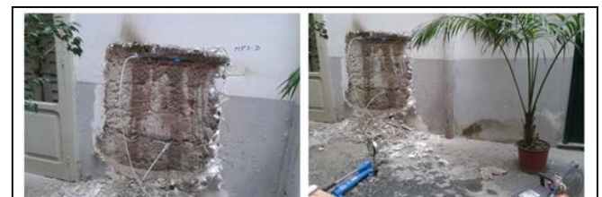
Figure 11. Flat jack test on the ground floor wall
