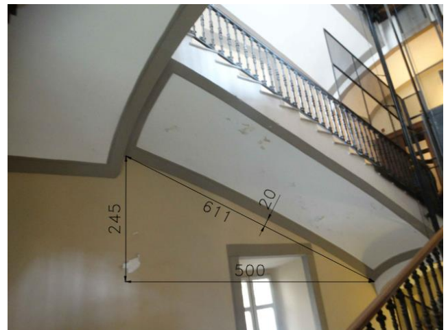
Figure 34. Roman-style rampant staircase and dimensions
