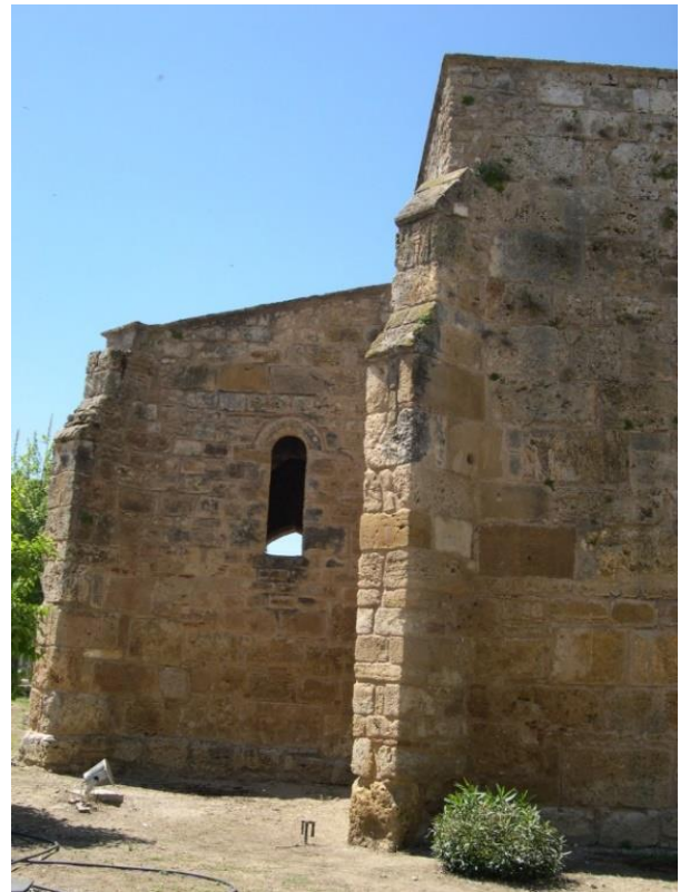
Figure 4. The diagonally laid pier buttresses at the exterior of the apse
