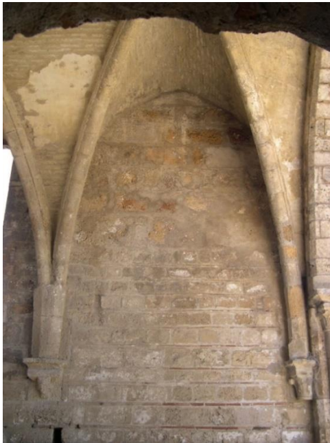
Figure 5. The ribs and springings of the vaults
