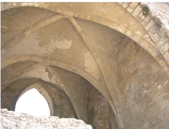
Figure 3. The ribbed vaults of the apse
