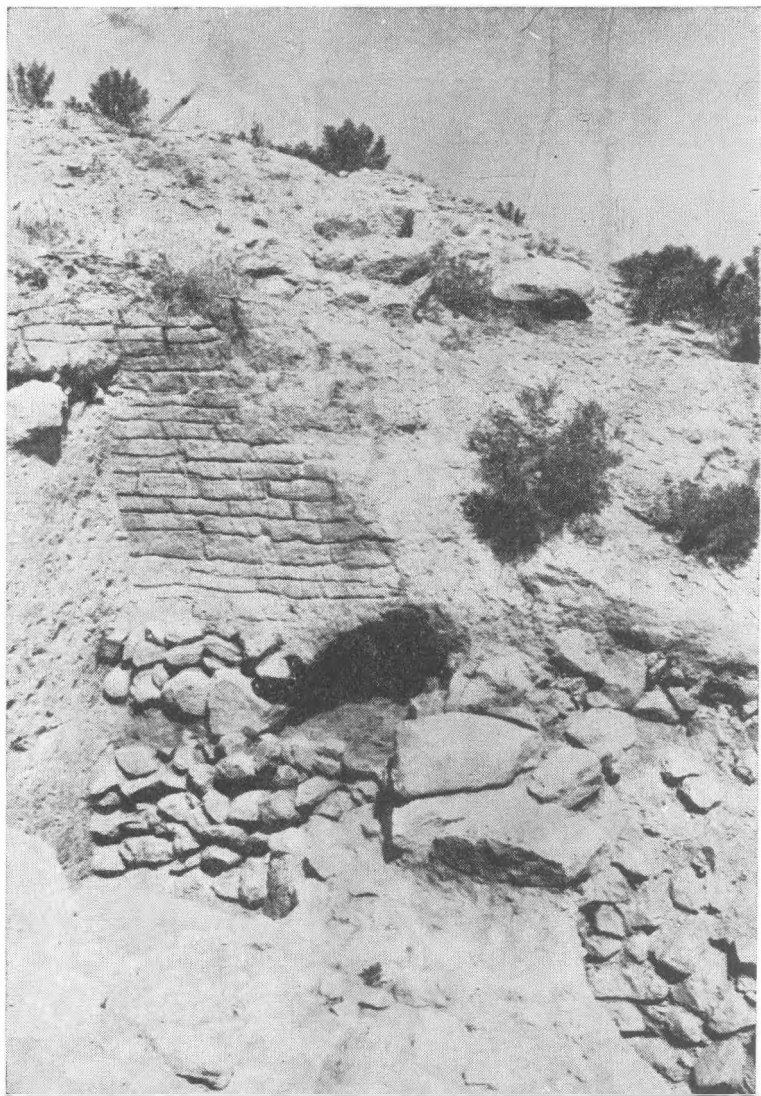
Fig: 3. The two defence walls in the western zone
