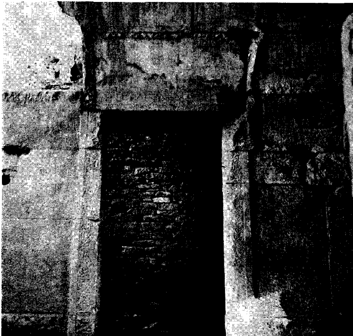
5 Theatre. Central vaulted tunnel of the stage building with door (cf. lintel inscription) communicating with side chamber,
