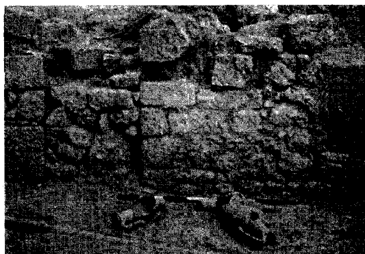
Fig. 58 — Roman House, blocked doorway indicating change in plan.
