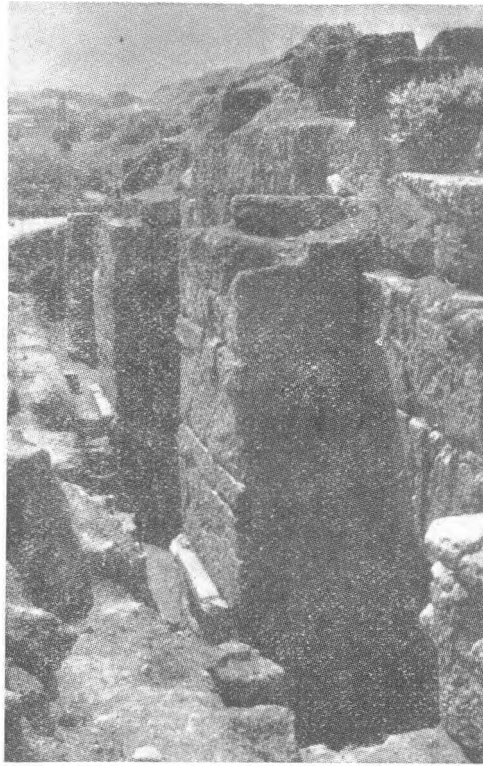
Fig. 19 — Building "CG", east facade after excavations of 1958, from north
