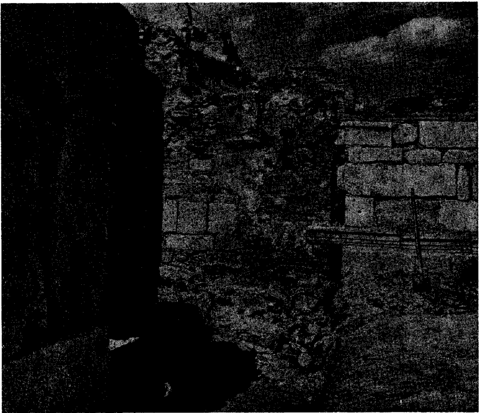
Fig. 29 Theatre. Stage blocking wall. Dismantled portion near north parodos and Archive Wall.
