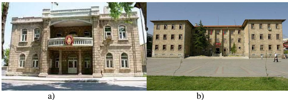
Fig. 3. Köfke stone application in Isparta province a) Garrison building (URL-5), b) Government building (URL-6)
