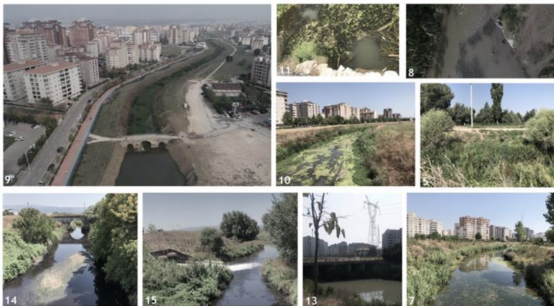
Figure 3. Photos from Problematic Areas, Ayvali Creek
