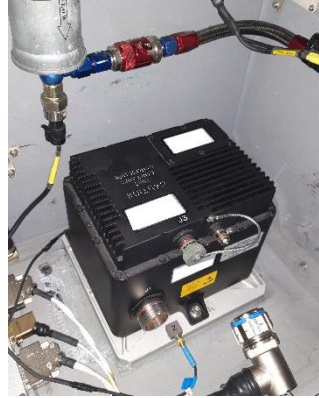
Figure 16. INS Mounted Test Setup for Installation Design Alternative 2
