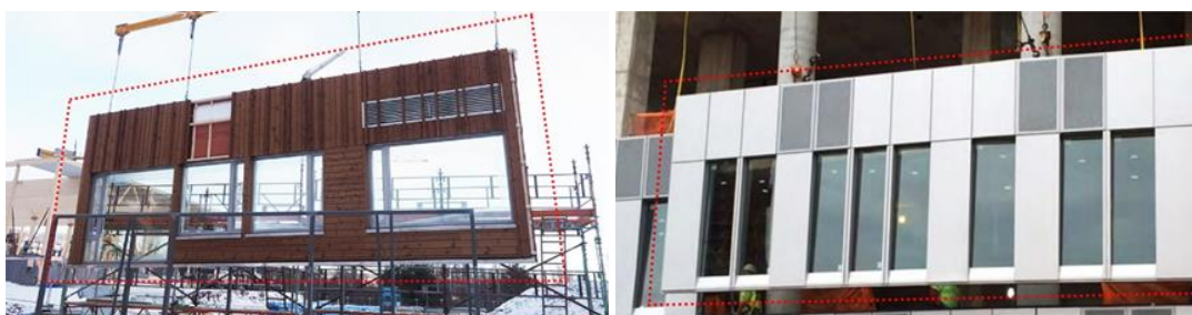
Figure 6. Examples of frame prefabricated facade panels based on wood and metal (Cornell Tech NYC; Jørn Hindklev, 2022)
