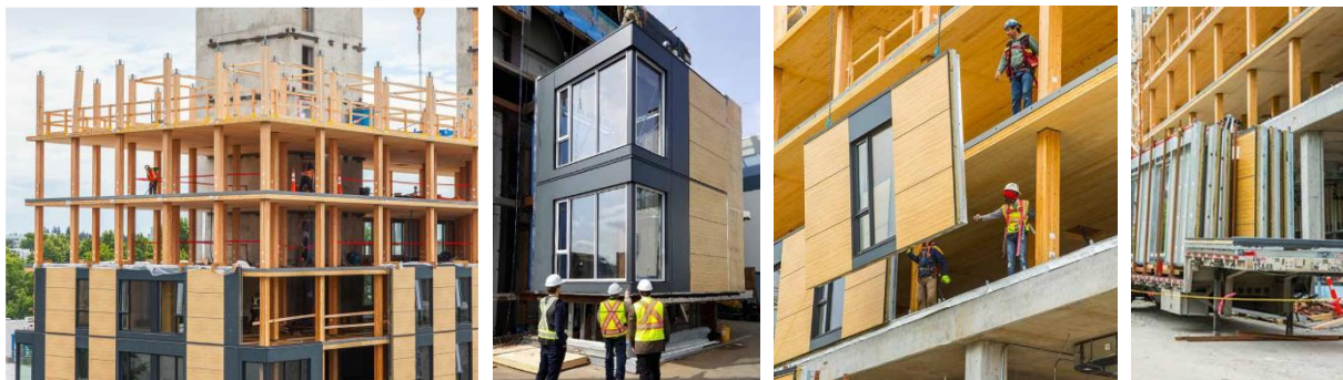
Figure 1. Example of prefabricated facade panel (Brock Commons Tallwood House) (NaturallyWood, 2017)
