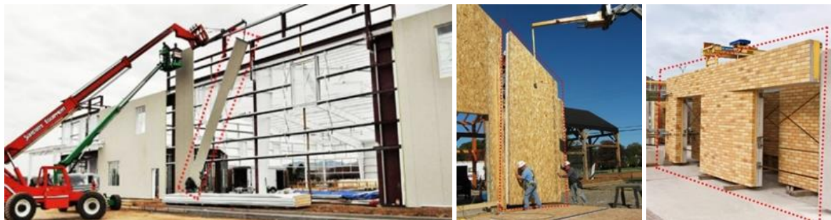
Figure 5. Examples of sandwich prefabricated facade panels based on metal, wood, and concrete (FIP; Sunny Pavilion; The Lansdowne, 2022)
