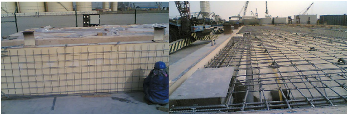
Figure 2. Phases of mold preparation
