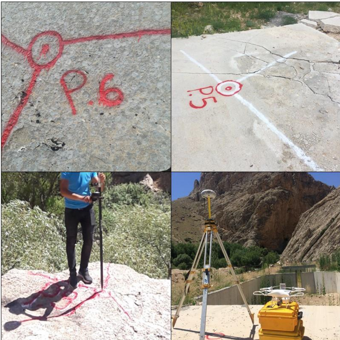
Figure 3. Marking and measuring GCPs
