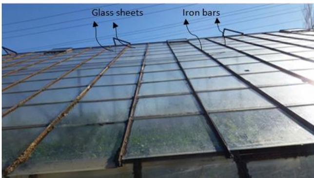
Figure 1. Glass greenhouse structure
