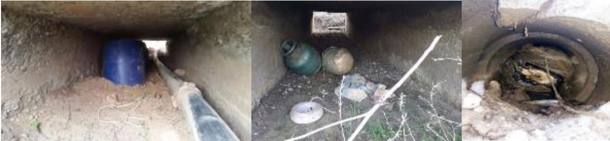
Figure 1. Images of HMEs planted and hidden in culverts [5–7]
