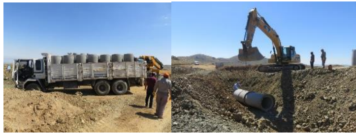
Figure 4. Concrete pipe culverts
