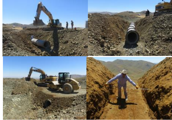
Figure 7. The installation process of the culverts
