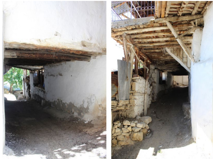
Figure 21. Gubuşlar Covering (Photo:Author)
