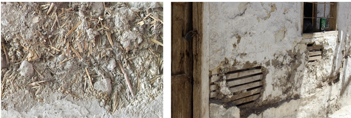
Figure 13. Wall Plasters (Photo:Author)
