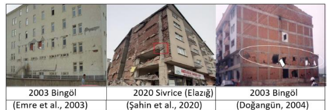
Figure 4. Moderate damaged RC buildings
