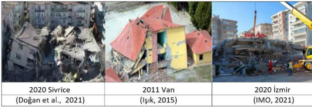
Figure 7. Destruction of (Grade 5) RC buildings
