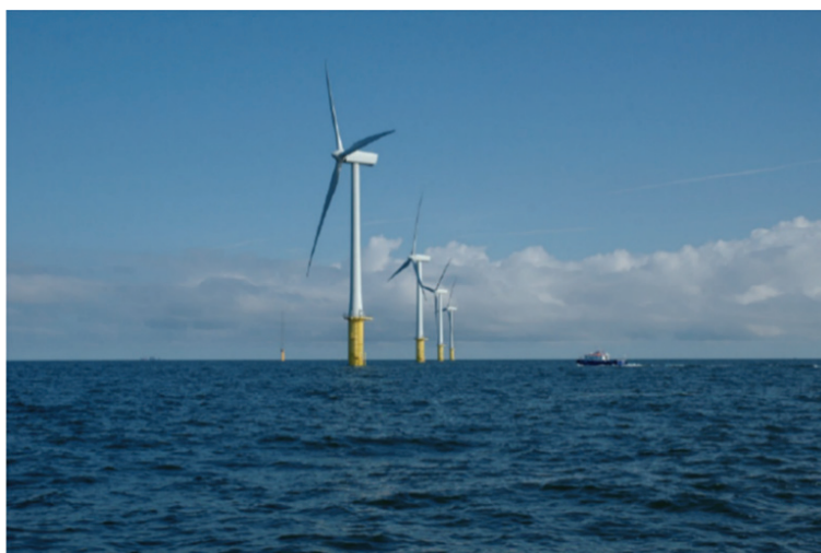
Figure 8. Vestas V80 - 2.0 offshore wind turbines of the North Hoyle wind farm (Hau, 2013).
