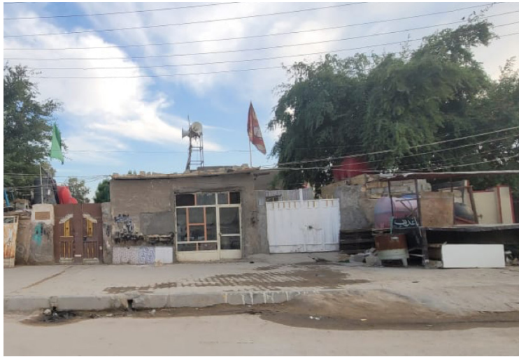
Figure 4. A housing in Karbala City (photo credit: A. Kadhim)
