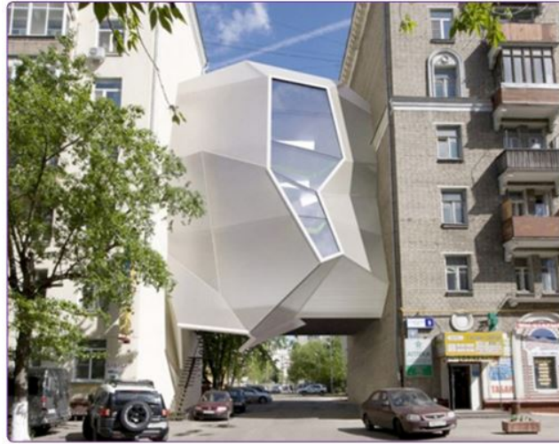
Figure 9: A parasitic structure clinging to two opposite idle façades (Yorgancıoğlu & Seyman Güray, 2018)
