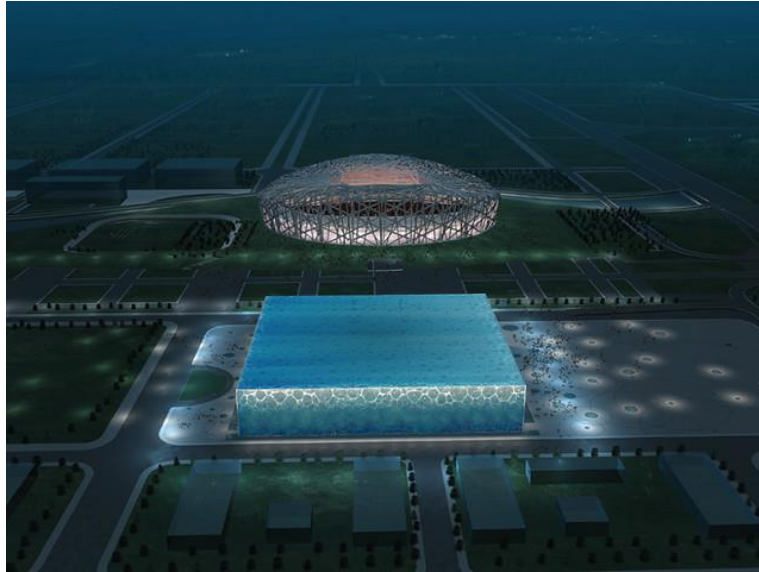
Figure 8. Water Cube National Swimming Centre, Beijing, PTW Architects. In the design of the building, a structural order derived from the soap bubble geometric algorithm was created [25].
