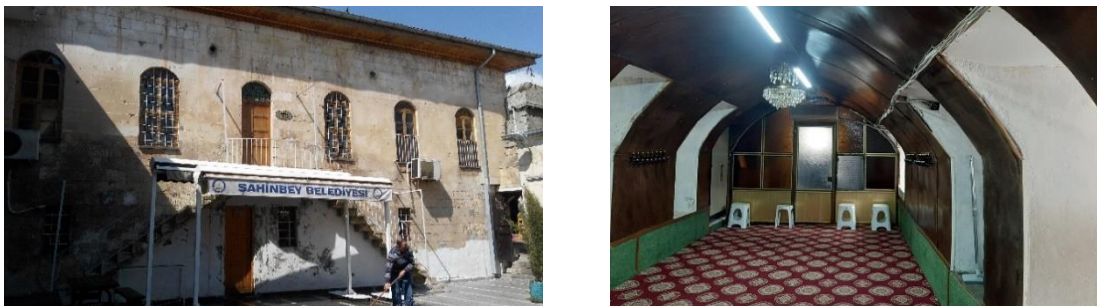
Image 11. Bekirbey Madrasah entrance facade (left) and interior view (right)
