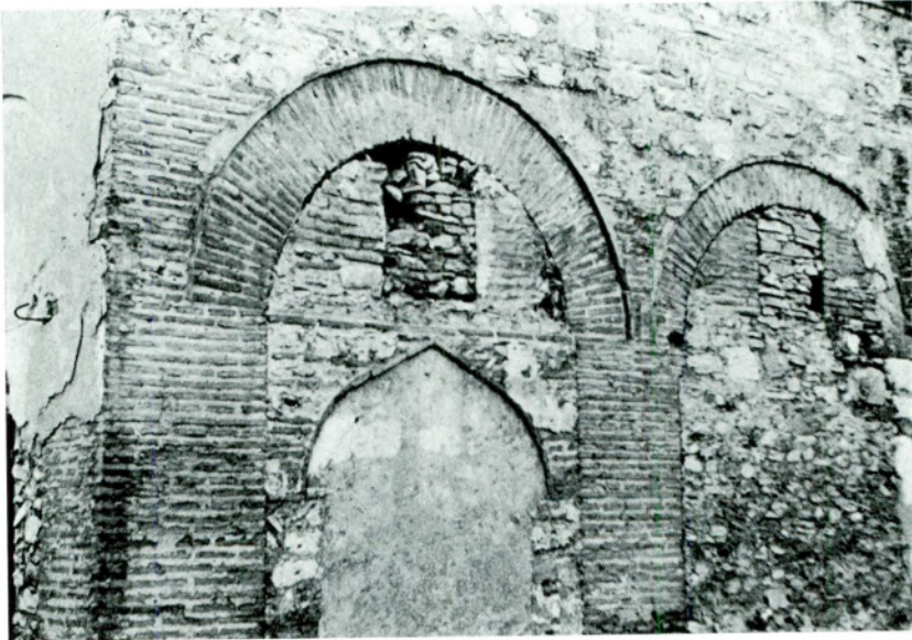
Fig. 4 — Stara Zagora, Hamza Bey Mosque, detail of walled-up gallery
