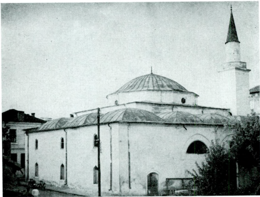
Fig. 9 — Jambol, Eski Cami. General view. Notice the enclosed “son cemaat yeri” and its walled-up arches
