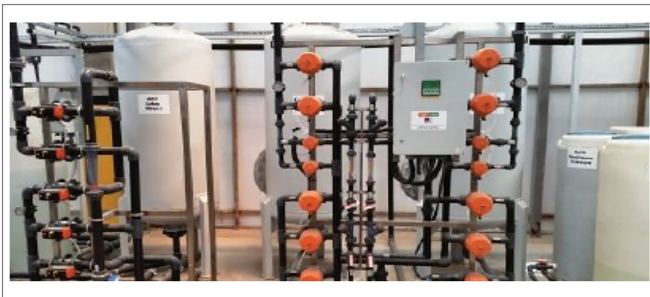
Figure 2. Demineralisation unit in Facility-A.
