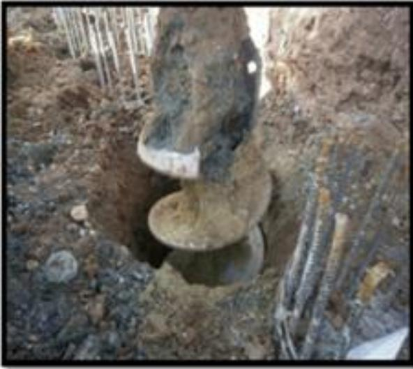
**Figure 7.** Phase 1 Bored pile construction
