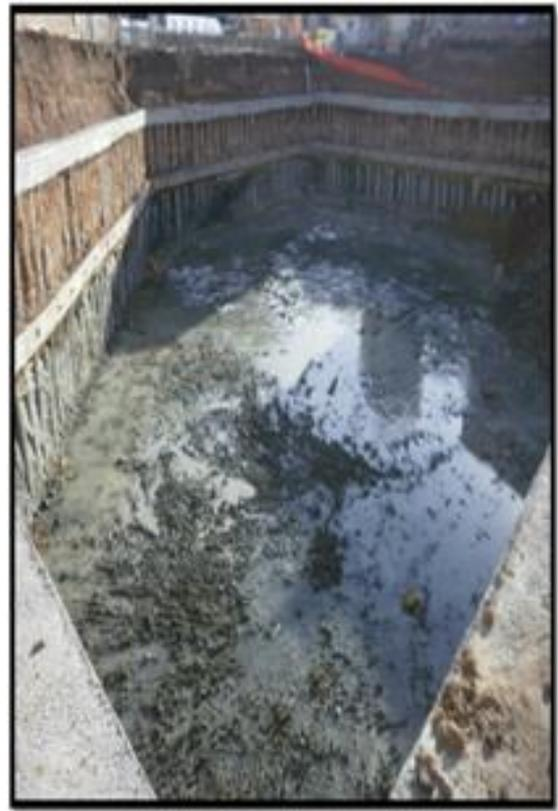
Figure 12. Phase4-Excavation completed
