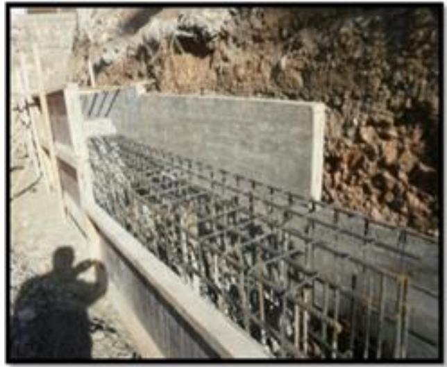
**Figure 8.** Phase 1 Capping beam construction
