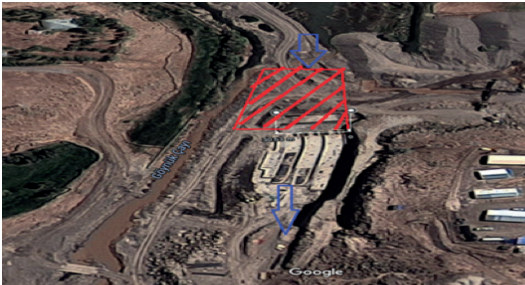
Figure 25. Existing reservoir for Saf HPP (3 m deep-40 ha)
