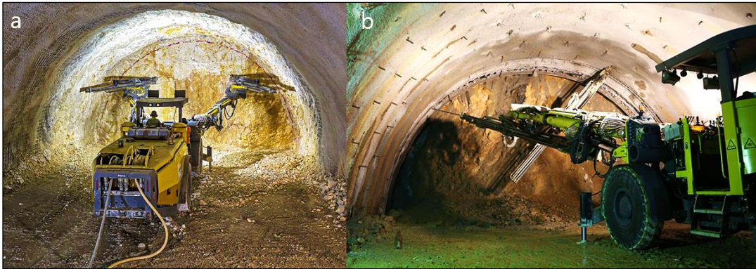
Figure 13. A view from double (a) and single (b) arm excavators digging Kirkdilim tunnels 32
