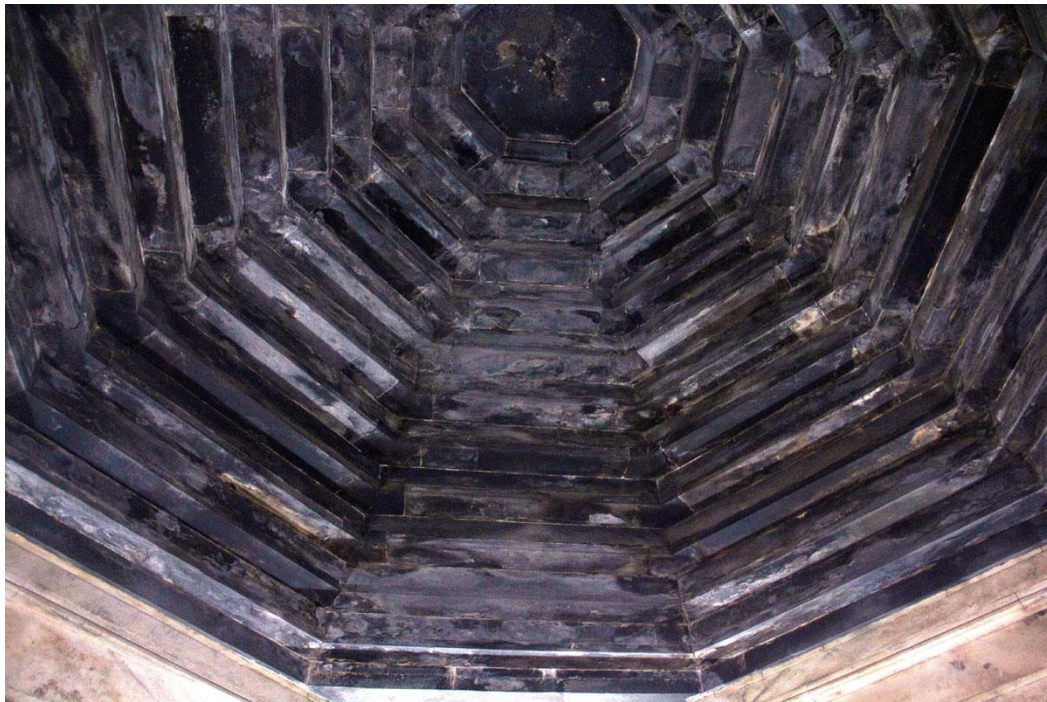
Ceiling internally with corbelled technique, Source: Shajjad Hossain, 2015
