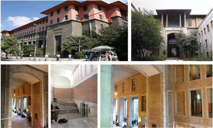
Figure 3. Facade and indoor photographs of the building at the Faculty of Science and Letters of Istanbul University (Bozkurt et al., 2019).
