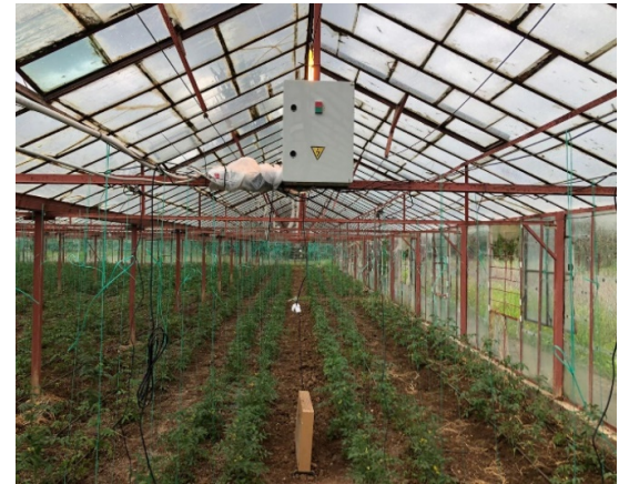
Figure 4. Fully functional irrigation system implemented in the test site
