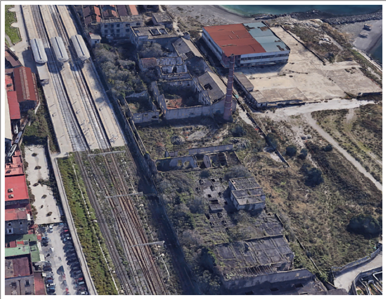
Figure 5. Case study area: The former industrial area Corradini, Naples.
