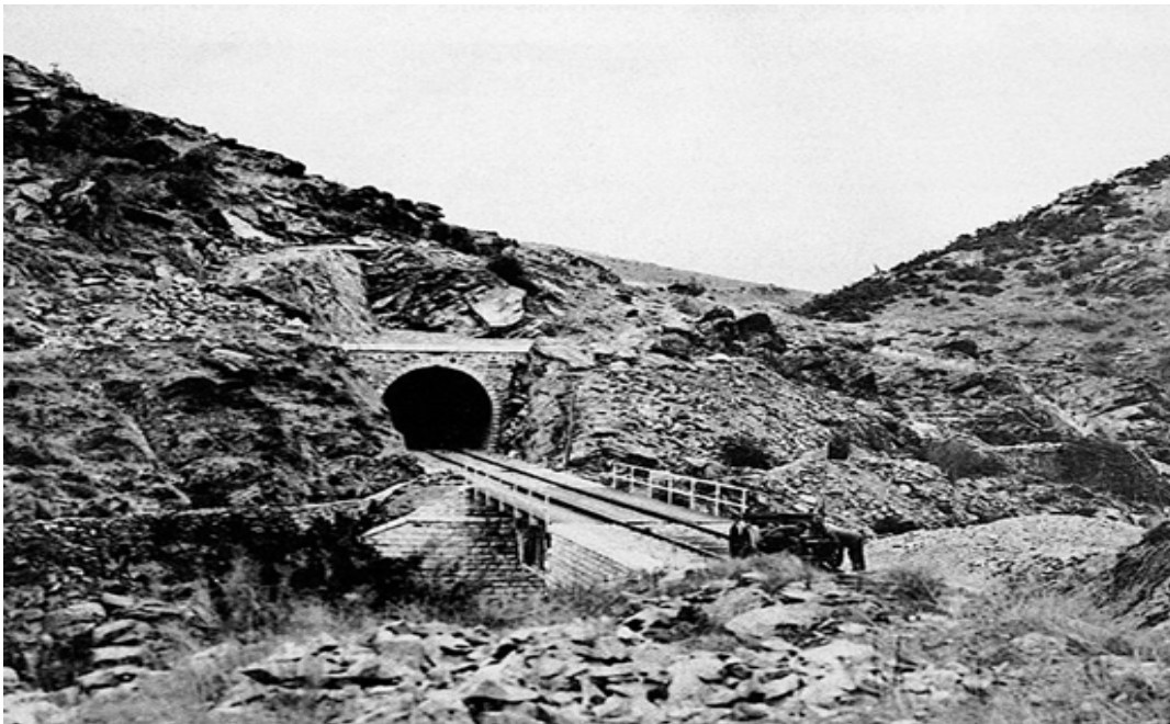
Figure 2: Rumeli Railway, An Unconstructed Tunnel on Thessaloniki-Istanbul Line
