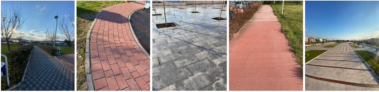
Figure 32. Flooring materials (Original, 2022)
